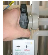
Three-way valve drain position
